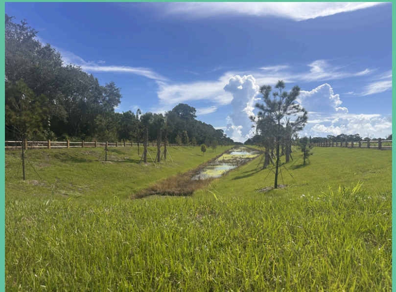
Sheraton Plaza Stormwater Treatment Area (STA)
